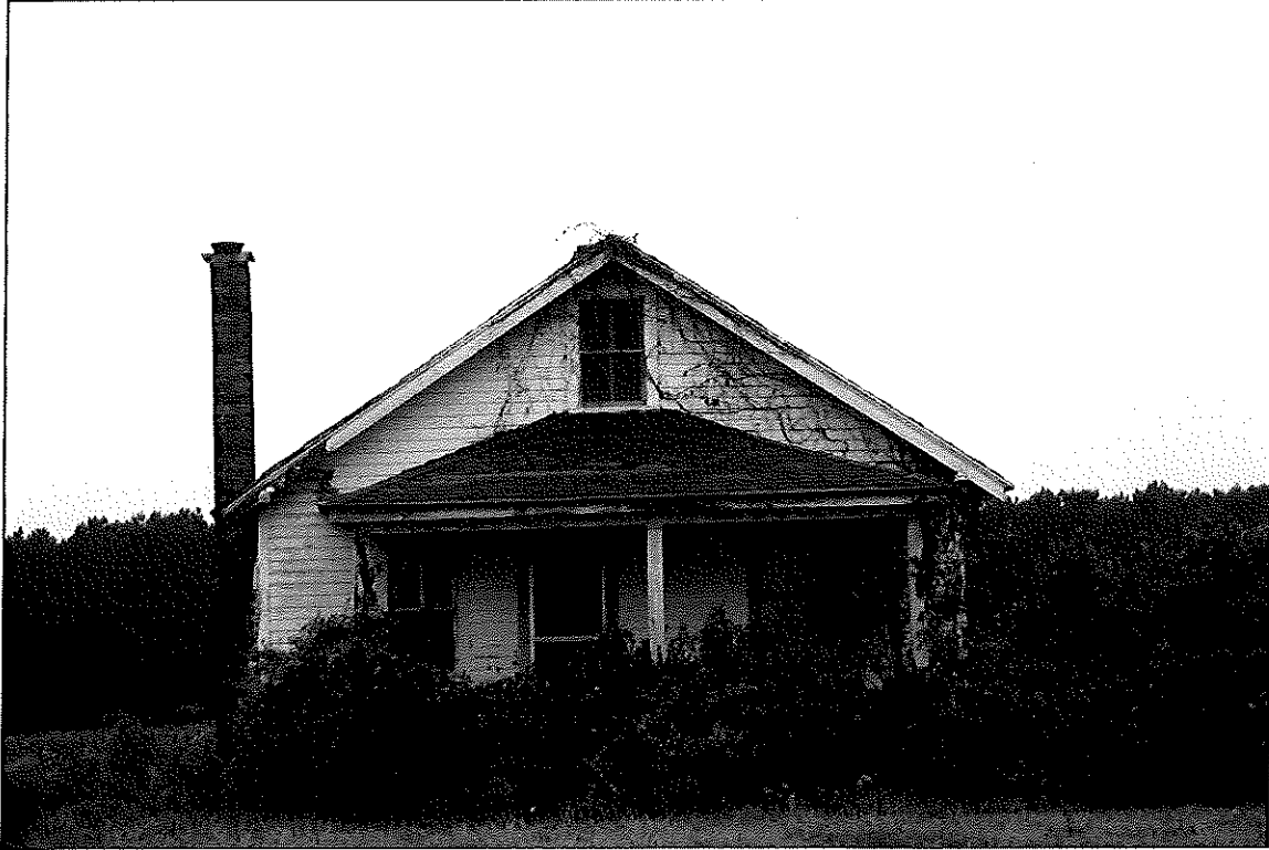
54. House, N side US 17, roughly across from #55 (No longer extant as of January 2005)
