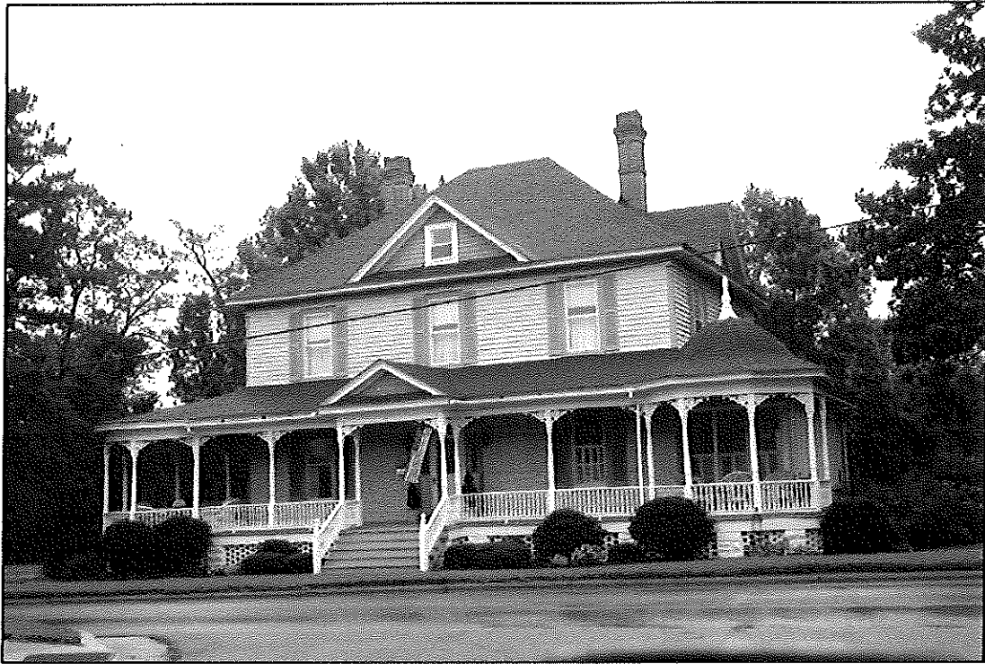
30. Adenine Cobb House, King Street
