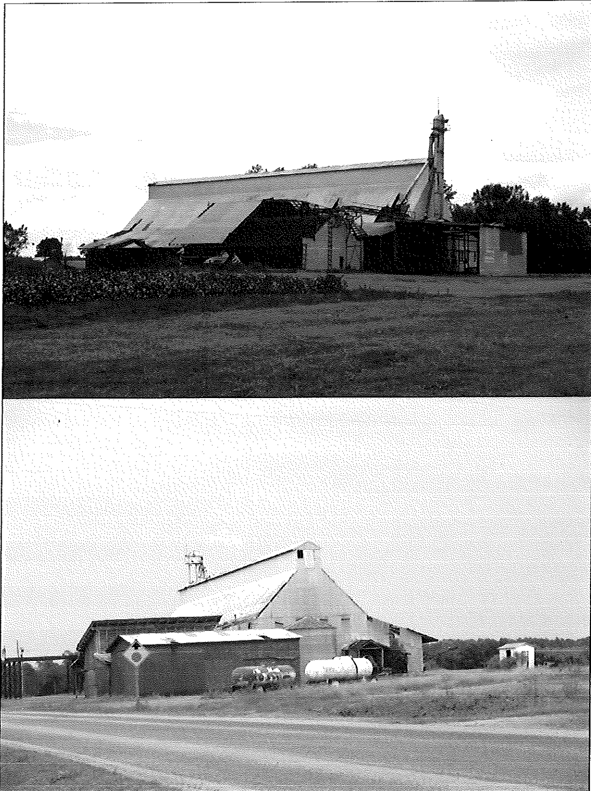
16. Bell Brothers Inc. Peanut Plant Complex, SW corner US 13 and SR 1100 (top shows view of southeast corner of complex from US 13; bottom shows view of northwest corner of complex from SR 1100)
