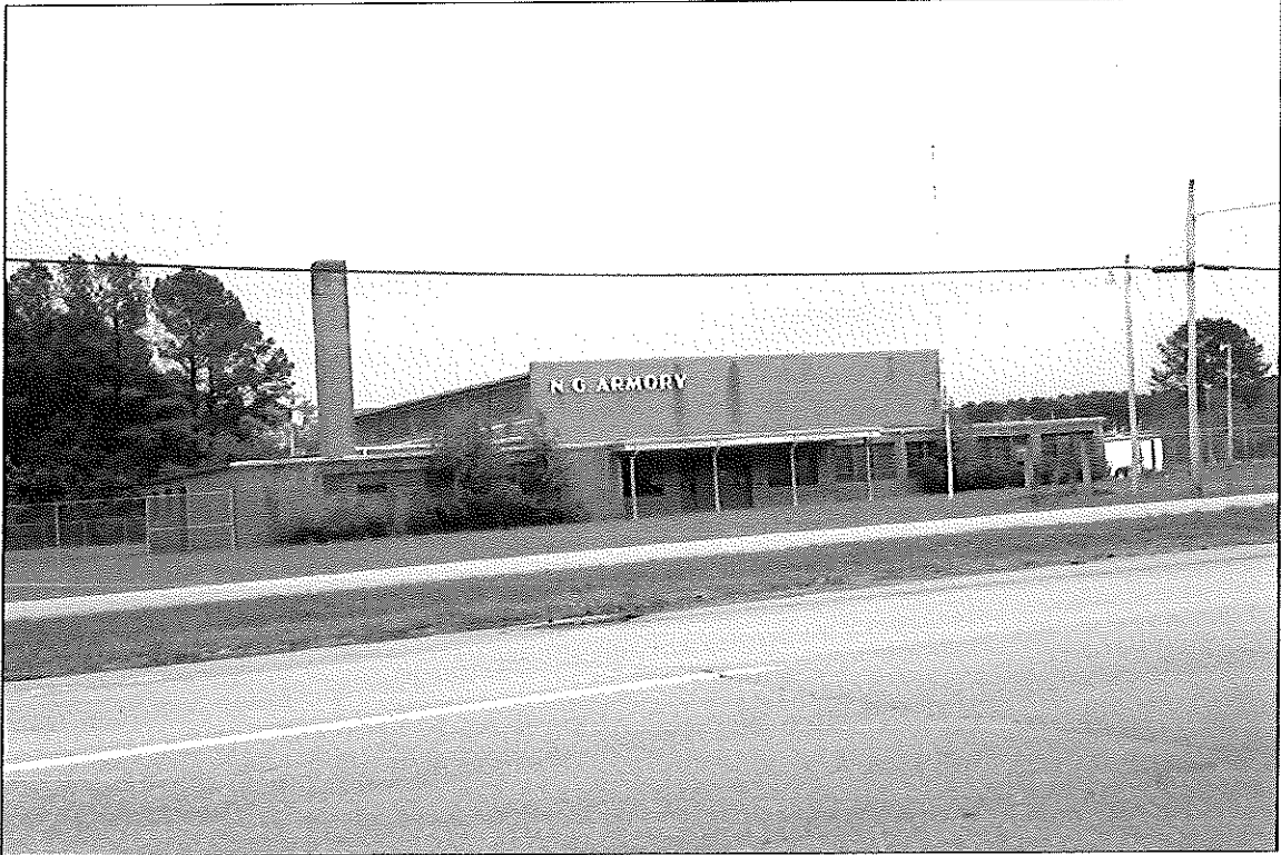
1. National Guard Armory, E Side US 13 (demolished as of January 2005)
