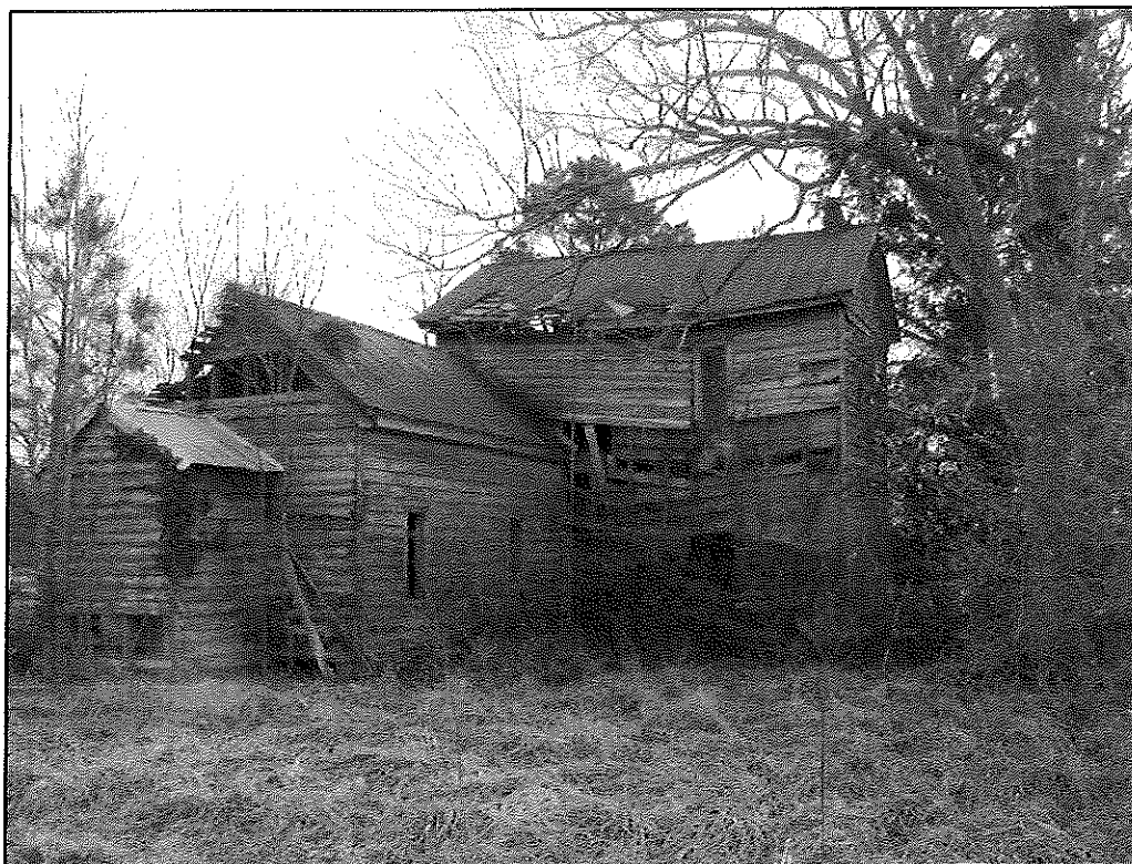
Figure 32. Harden Tenant House, rear view
