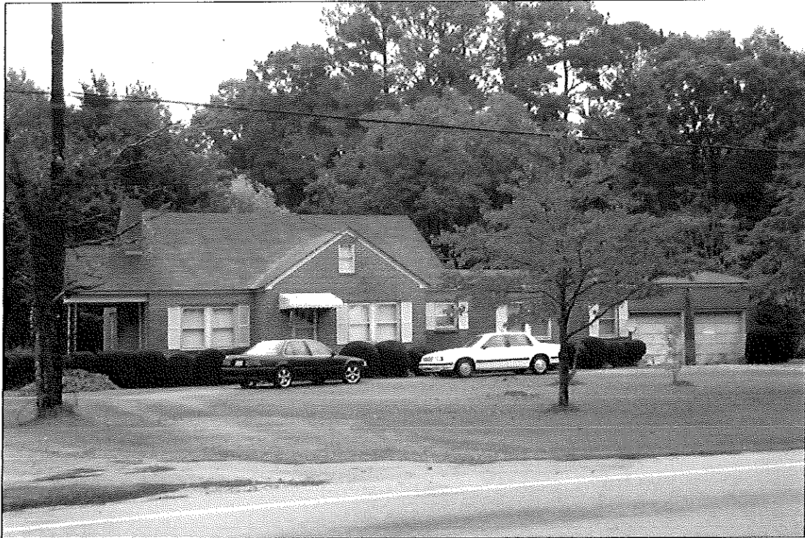
22. House, 1205 Sterlingworth Street (NC 308)
